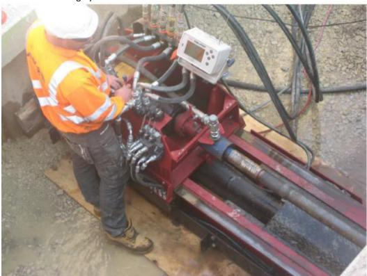
All Hydraulic operation of the Pit Launch directional drilling rig
