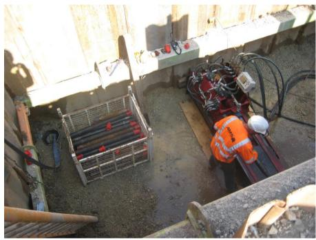
AMS No-Dig's Pit Launch directional drilling rig in place ready to start drilling
