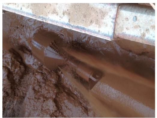
36 inch steel pipe entering the bore
