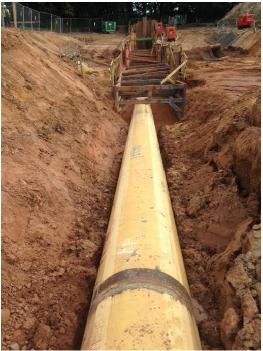
36 inch steel Pipe at rig side following installation
