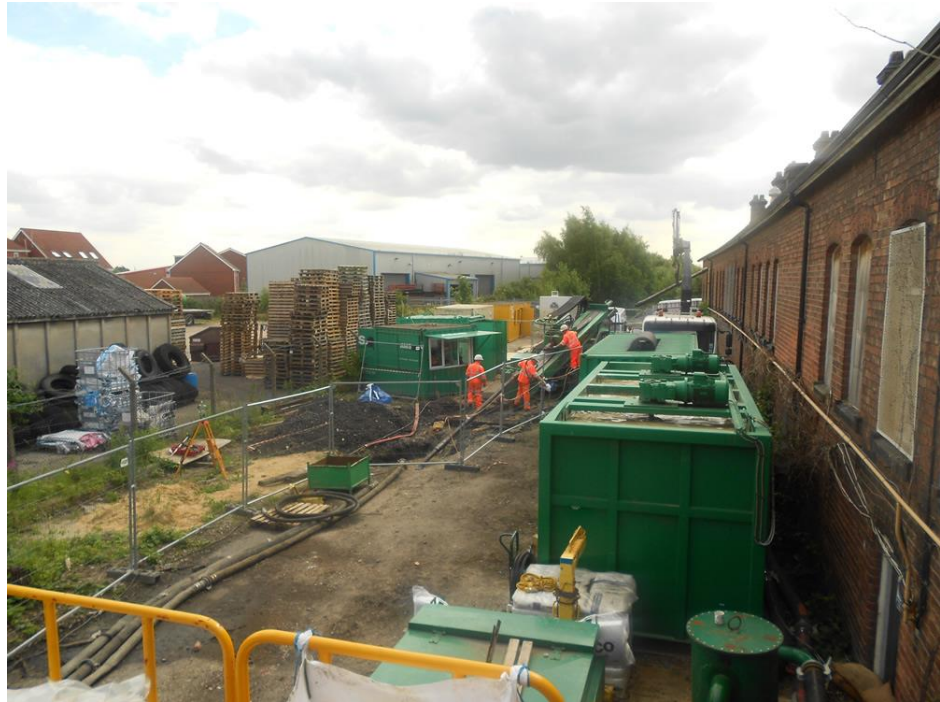
The compact drilling site at Selby
