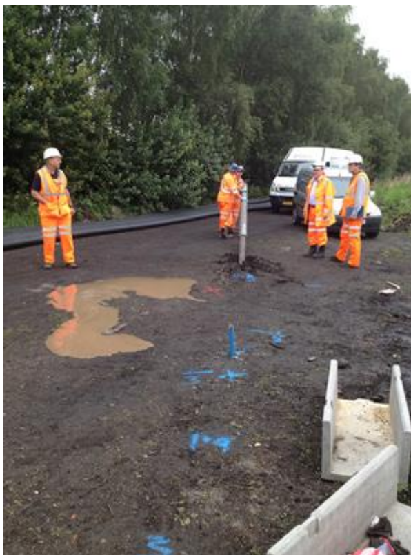
The exit point showing the accuracy of the gyro steering tool
