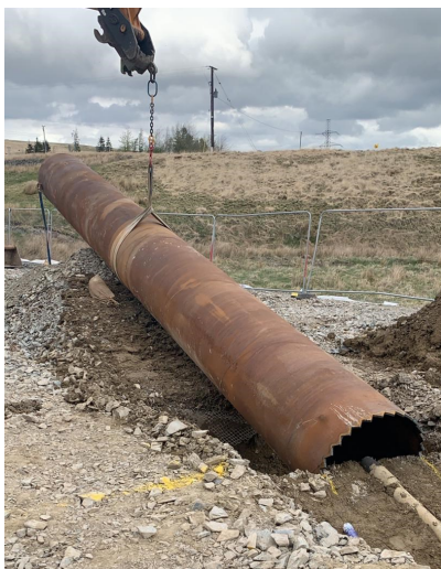
Casing pipe in place
