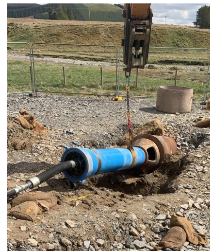
Casing pipe installed
